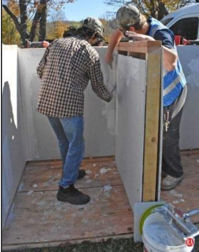
Charles Fields, right, of Enfield, guides Owen Crumlich of New Milford at the hanging and taping station during the Touch A Trade event Saturday on the grounds of Connecticut Antique Machinery Association in Kent. All of the presenters donated their time and admission was free. Lynn Mellis Worthington Republican-American
